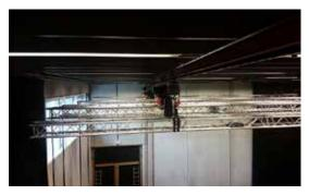
7x truss Prolyte X30V (square 30cm x 30cm) 13m, each on 2 motors Prolyft PLF-11 (500kg). Maximum free heighth under the trusses: 6m90. The motors hang on trolleys, so they can be moved in the length of the studio. Motor control: maximum 4 motors can move at the same time.
