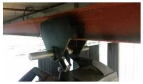
On the ceiling of the studio, there are 6 I-beams, in the length of the studio, with a maximum point load of 500kg. Free heighth under the I-beams: 7m90. Under the I-beams, there are trol-leys (manually controlled).
